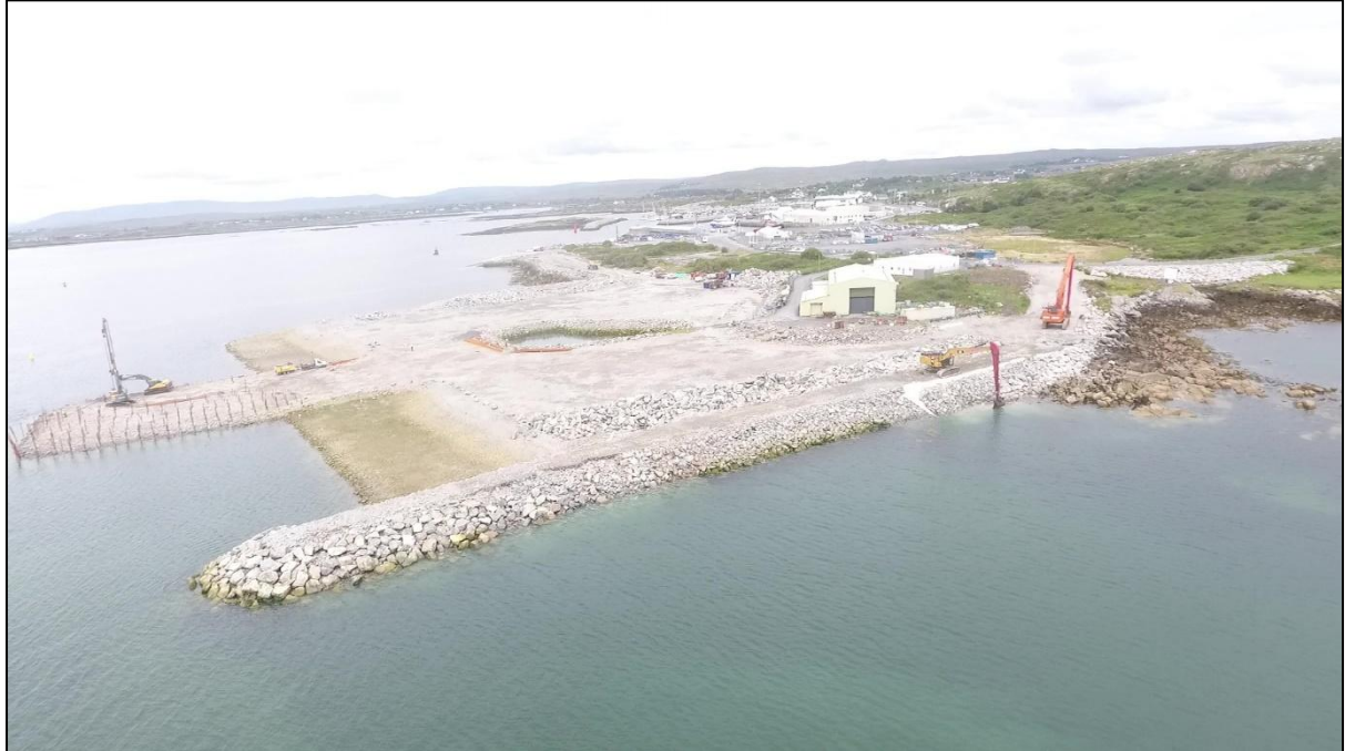
Figure 4 Development site status 10 th July 2023
